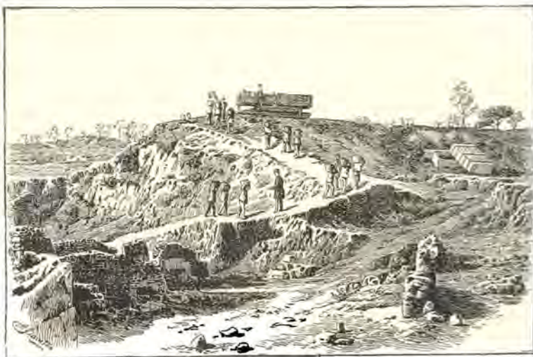
BOYS CARRYING SOIL FROM THE EXCAVATIONS.
