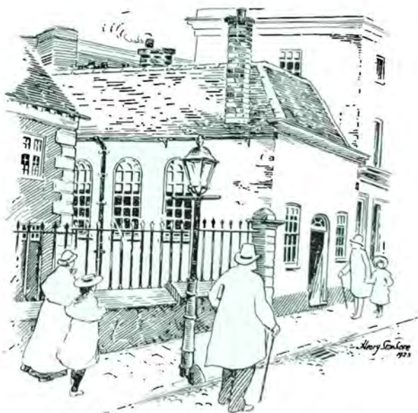
The Friar Lane Meeting House, Nottingham
