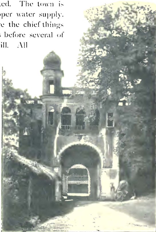
OLD GATEWAY AT PATNA. Entrance to Hospital Grounds.
