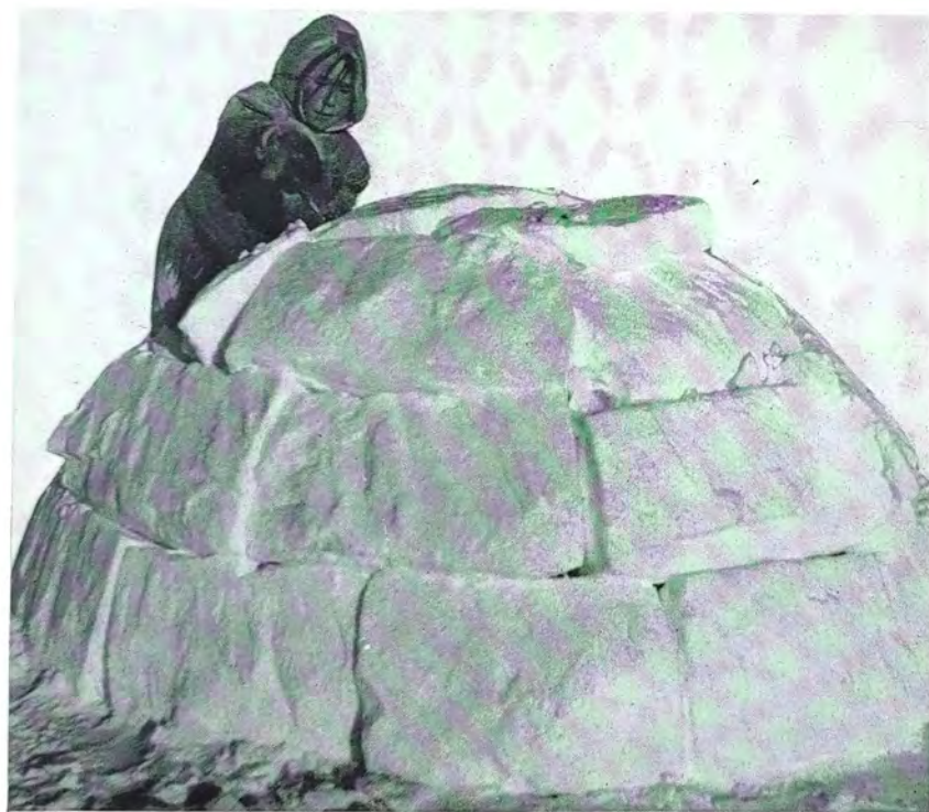
The very last job is chinking the igloo. The chinks are filled with soft snow to make the ice home windproof
