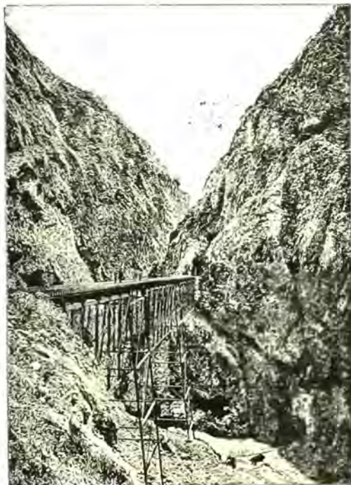
THE CHAUPICHACA BRIDGE ON THE OROYA RAILWAY, PERU. ANDES SCENERY.
