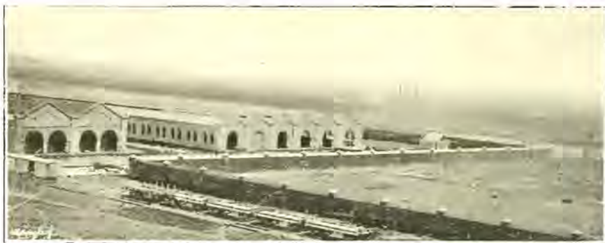
CENTRAL ARGENTINE RAILWAY WORKS.
