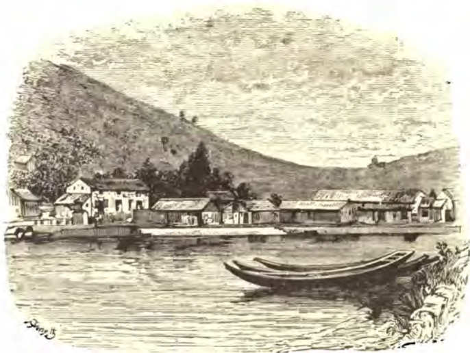
MOH-TS-IN, C.M.S. STATION ON THE EASTERN LAKE.
