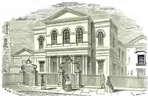
NEW PARK STREET CHAPEL.
