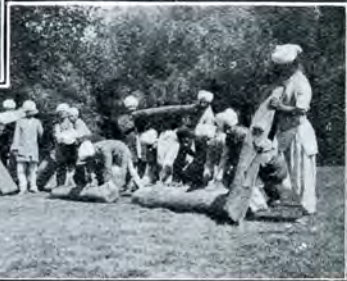
Carrying Logs for School Building
