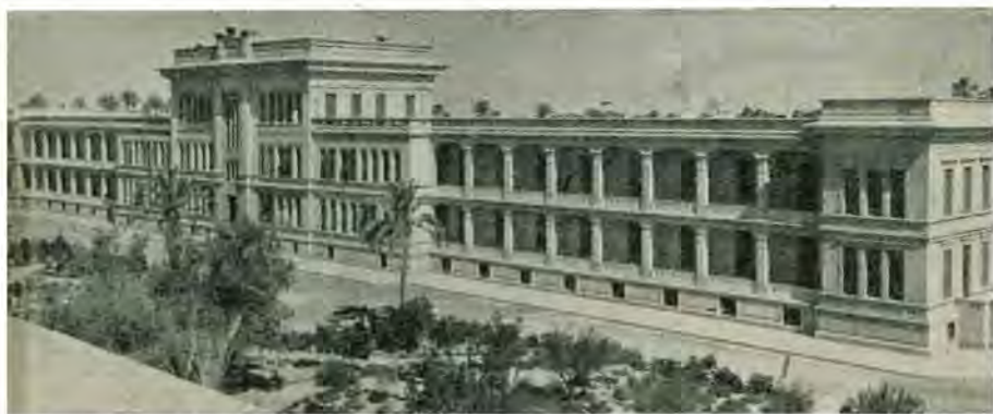
COLONIAL HOSPITAL, TRIPOLI
